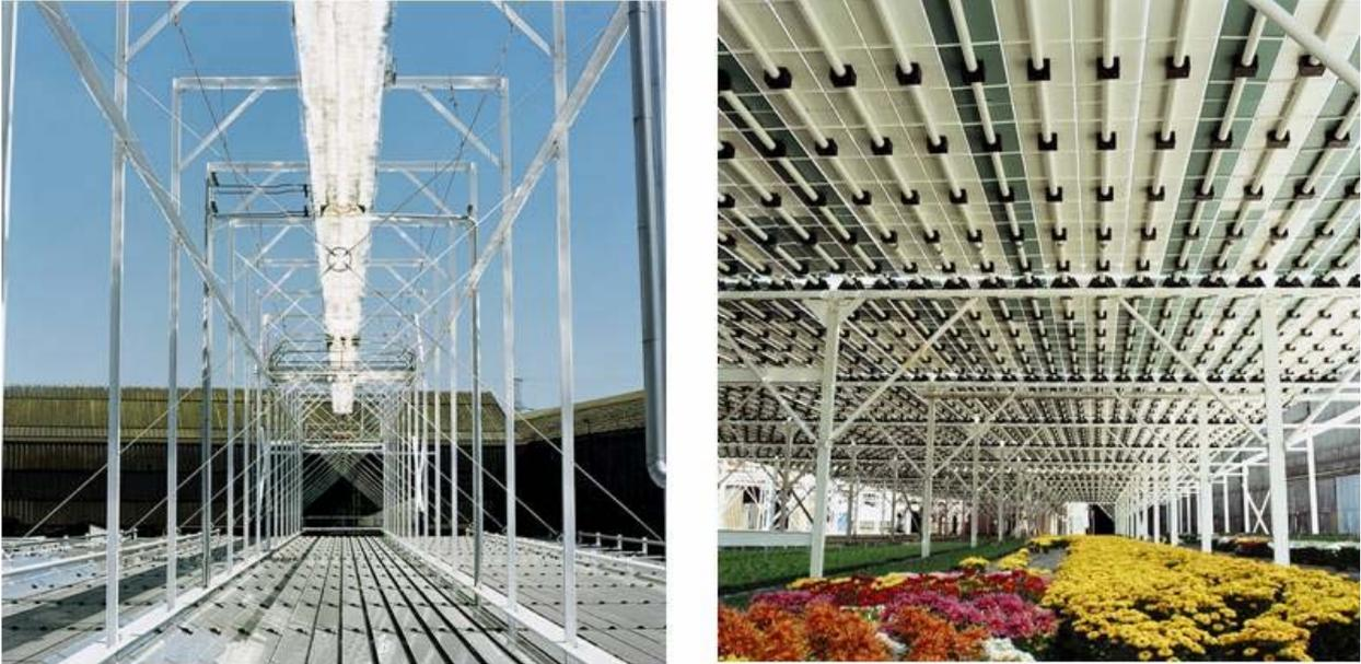
Figure 2: Concentrating solar collectors with parabolic trough mirrors to reflect the sunlight to the absorber pipe.
