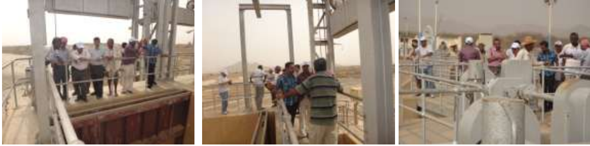
Photos from Wadi Mawr Main structure visit
