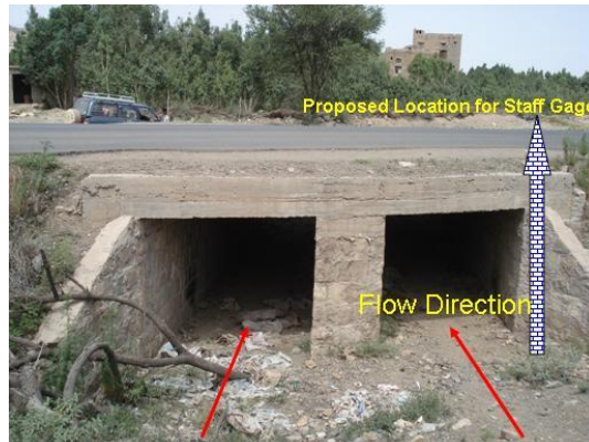
Figure 6-38 Proposed location for staff gage and data logger instrument (arrow with brick pattern) upstream of crossing structure at Wadi Al-Foros outlet
