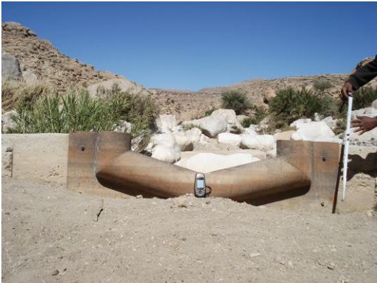
Figure 6-102 Existing V-Notch weir at Wadi Al-Kharid
