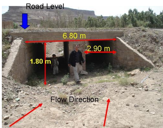
Figure 6-33 Dimensions of culvert openings
