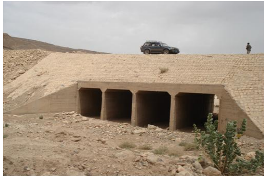
Figure 6-62 Upstream view of the crossing structure
