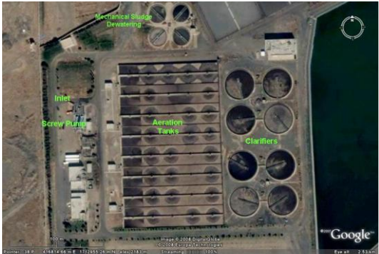
Figure 6-112 Aeration basins and trickling filters of Sana'a WWTP
