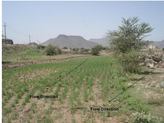
Figure 6-75 View of the upstream area in front of the culvert
