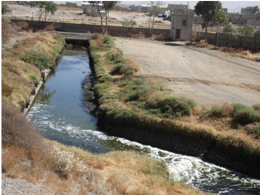
Figure 6-122 Inlet point of Sana'a WWTP
