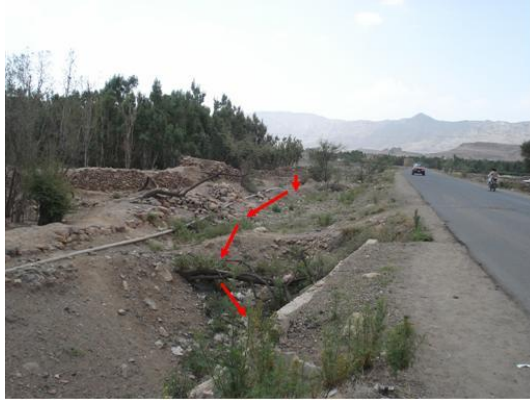
Figure 6-34 Upstream view from crossing structure
