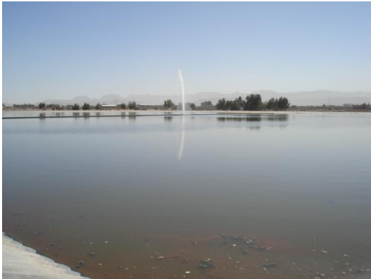
Figure 6-119 Polishing lagoon in Sana'a WWTP
