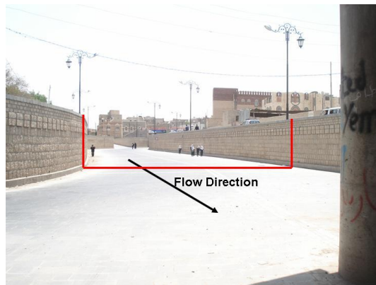
Figure 6-72 Upstream view from the bridge
