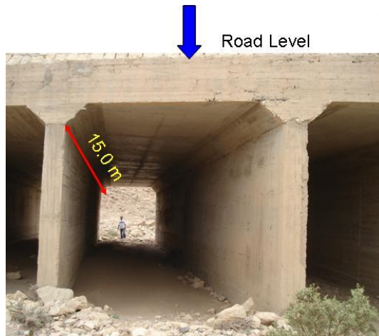
Figure 6-64 Depth of the culvert opening
