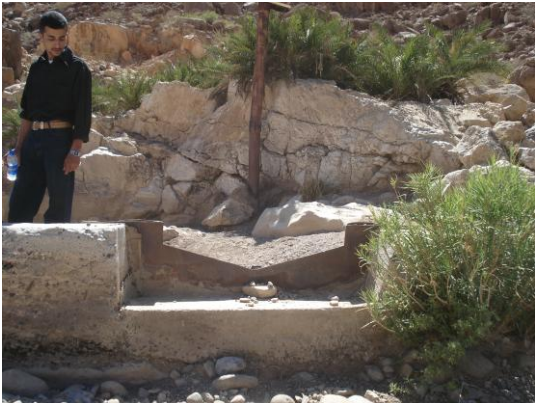
Figure 6-103 Backside view of the V-Notch weir at Wadi Al-Kharid
