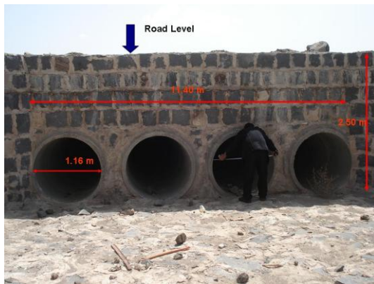
Figure 6-76 Culvert dimensions
