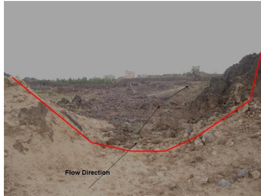
Figure 6-80 Upstream view of the main stream floodpath leading to the constructed reservoir
