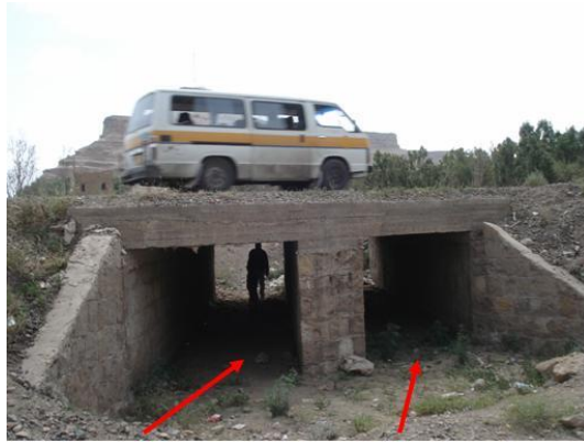
Figure 6-32 Culvert at the highway intersection near the outlet of Wadi Al-Foros. Flow direction is shown with red arrows. UTM coordinates for this location are UTME=426000 and UTM N =1710625, at an elevation of 2274 m (AMSL)
