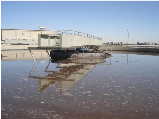
Figure 6-116 Trickling filters in Sana'a WWTP
