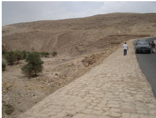
Figure 6-61 View of the highway and the downstream side of the floodway
