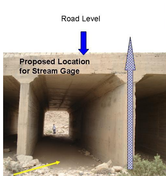
Figure 6-67 Proposed location for staff gage and data logger instrument (arrow with brick pattern) in the main stream of Wadi Khulaga floodway
