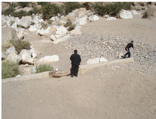
Figure 6-105 V-Notch weir and its concrete wings
