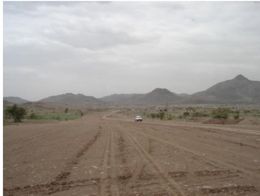
Figure 6-93 Road construction at the proposed monitoring location
