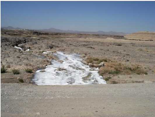
Figure 6-129 Downstream view of the Bani Garmouz road culvert
