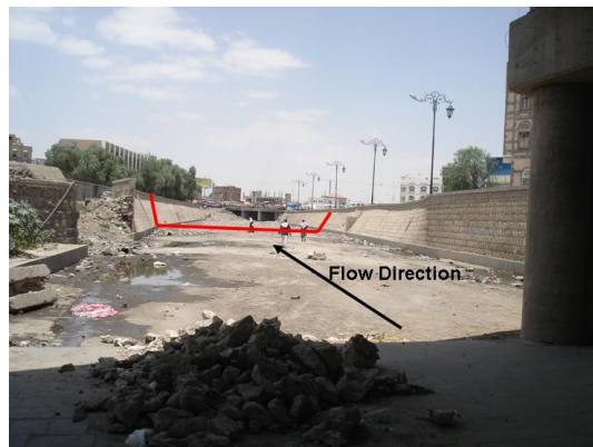
Figure 6-70 Downstream view from the bridge
