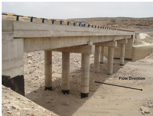
Figure 6-107 View of the bridge openings and piers
