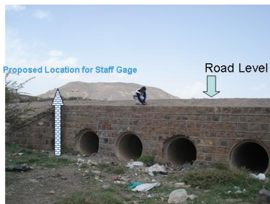
Figure 6-8 Proposed location for the staff and data logger instrument (wide arrow with brick filling)
