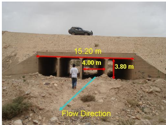
Figure 6-63 Dimensions of the box culvert
