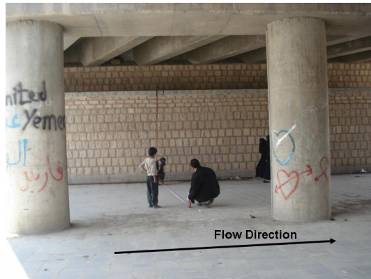
Figure 6-71 During the measuring of bridge dimensions
