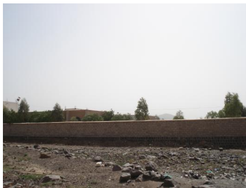
Figure A-4 Picture showing one of the schools that was selected for installing the new rainfall station Al_Shahied Abdelkhalek Azan School
