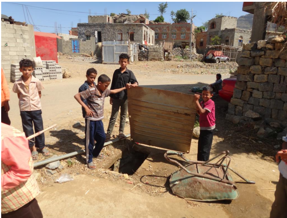
Figure 1. Water cistern filled by run-off from road-surface
