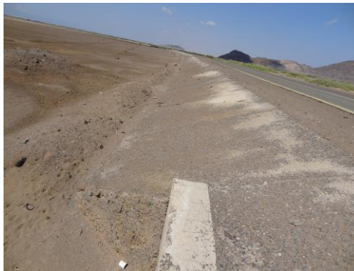
Figure 39. & 40. The embankment was protected by concrete and there is a small temporary bund to retain the water in the upstream (the potential is using gates in the culverts inlets).
