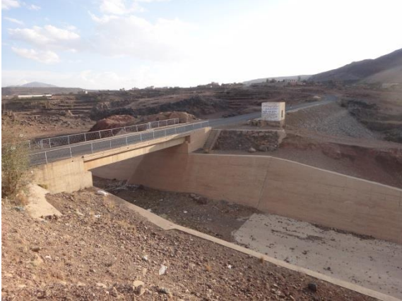
Figure 43. & 44. Road body used as recharge dam in asphalt road
