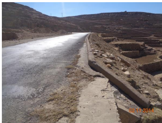
Figure 30. & 31. Erosion from uncontrolled run-off (left) and controlled road run-off (right)
