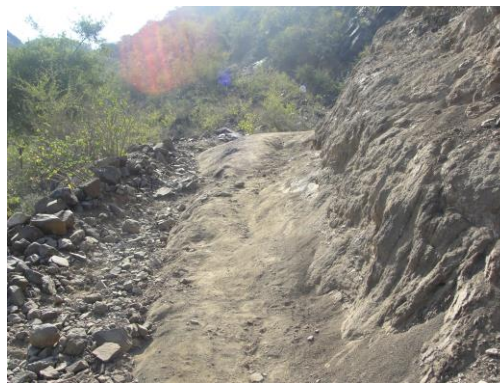
Figure 41. and 42 : Earthen roads risk developing into a flood path – proper design with rolling dips and spill overs required.
