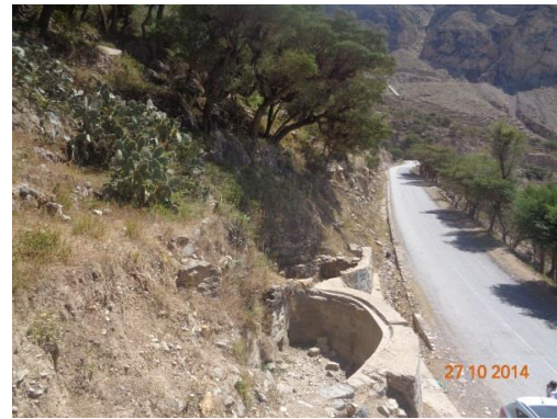
Figure 25. & 26. Pond storing spring water at down-slope accessed by a pipe (left) and spring water protection box up-slope (right)
