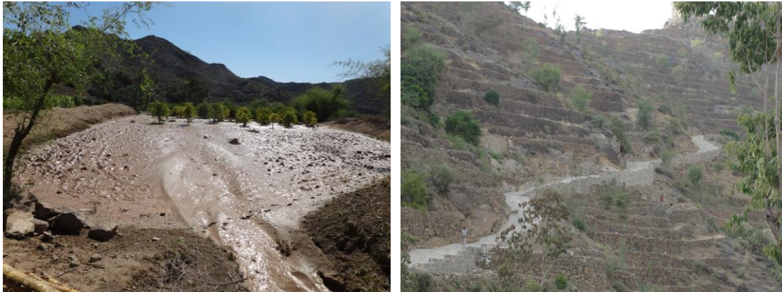
Figure 10 & 11. Direct irrigation from road surface and water harvested from side curbs
