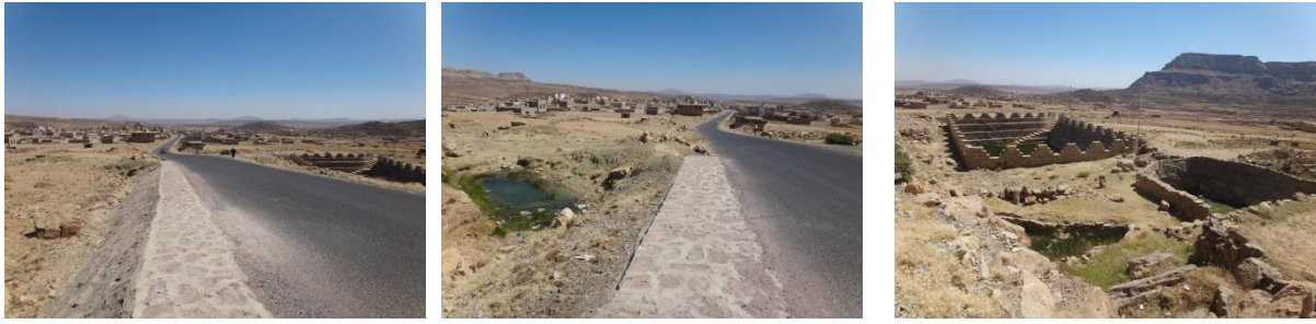
Figure 19. & 20. & 21. Road embankment (left) interferes with base subsurface spring flow; the intercepted water appeared on the other side (picture at the middle) of the spring flow point (picture at the right): by using a clever permeable road foundation this problem can be avoided.
