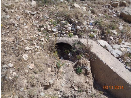
Figure 32. & 33. Blocked culvert inlets
