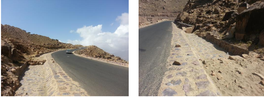
Figure 37. & 38. Temporary rock scour checks in a rip-rapped side ditches
