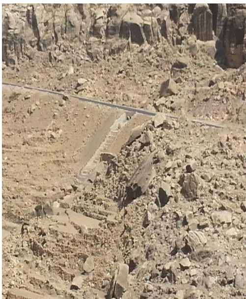
Figure 34. & 35. Lined road drains
