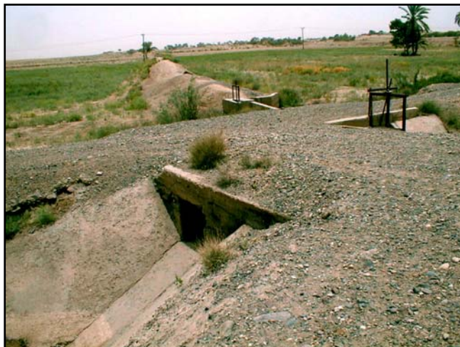
Ras Al Wadi, Secondary Canal Check Drop and Turnout, August 2002
