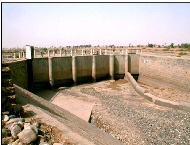
Faleg Weir Head Regulator & Scour Sluice Wadi Kabid
