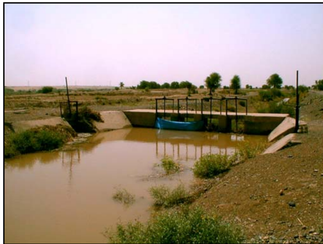
Al Arais Main Canal & Cross regulator at P26 Turnout, 12 August 2002
