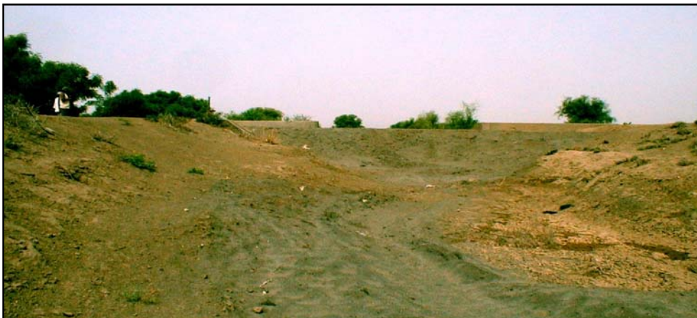
Yusufi Canal showing Sediment & Bund to Divert Flows to Outlets, 8 th August 2002
