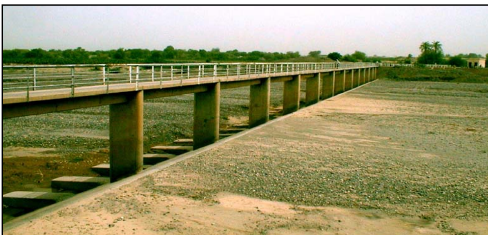
Weir 3, Main Weir Crest, 7 th August 2002
