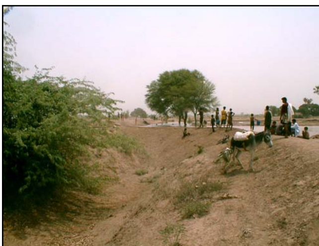
Ebry-Gerhazy CA. View of water distribution “channel” looking upstream. An earthen bund is diverting flow to upstream fields. Later, this bund will be cut releasing flow to downstream users.
