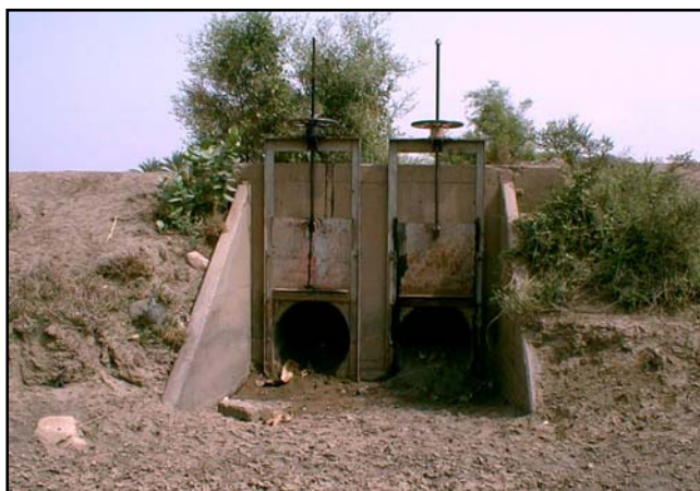
Gated Pipe Culvert Outlet from Yusfi Canal
