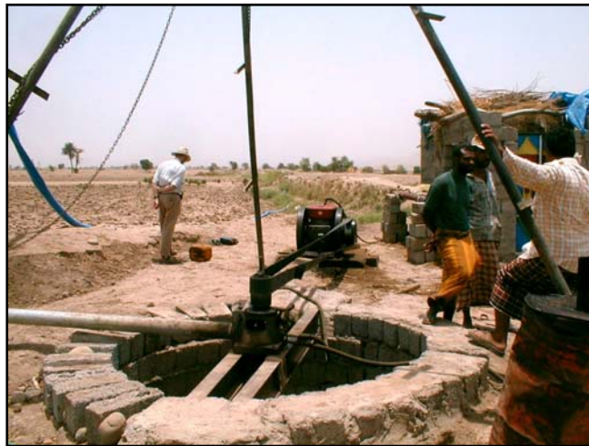
Pumped well in Al Arais Command Area
