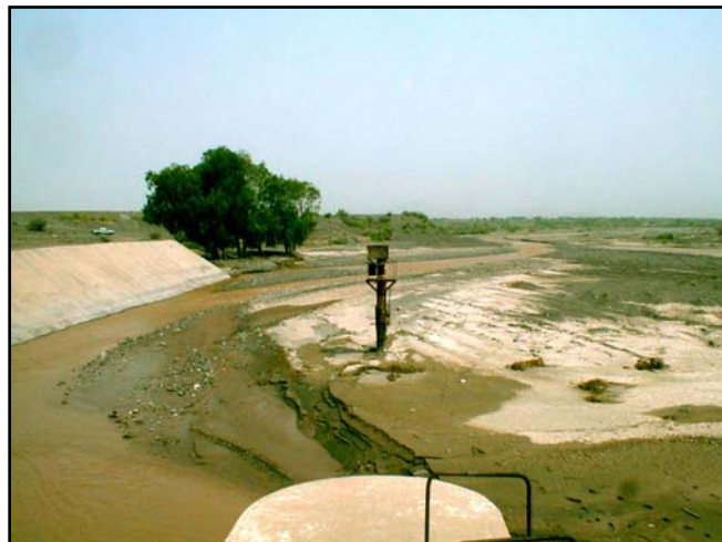
View upstream of Al-Arais Head Regulator showing (disused) Gauging Structure
