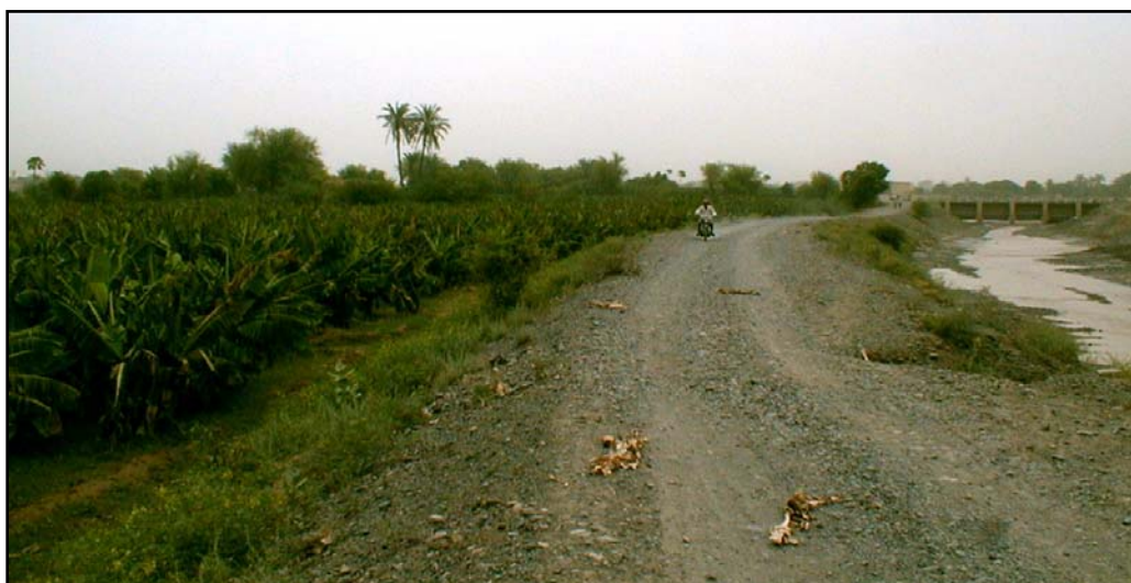
Mawi-Yusfi Canal, Looking Upstream to Weir 3, 7 August 2002
