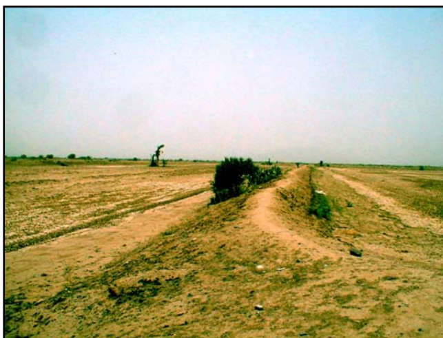
Al Arais CA showing Field Bund & Field Drop structure, 11 August 2002
