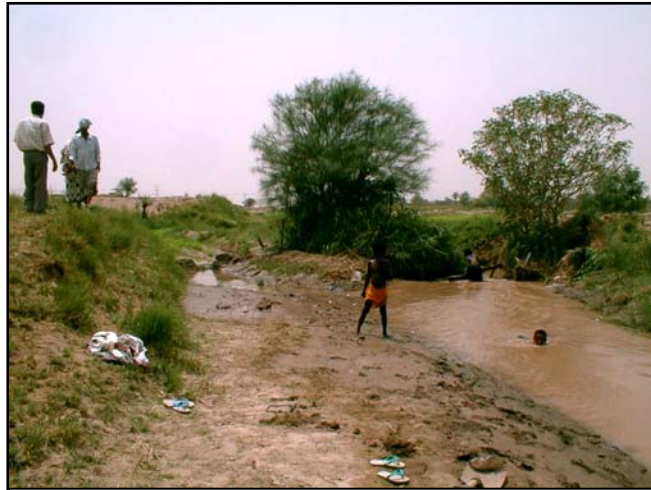
Small Traditional System, Primary Canal with “Stick & Earth” Check
