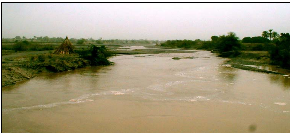
Weir 3 Looking Upstream from Left Side Head Regulator
