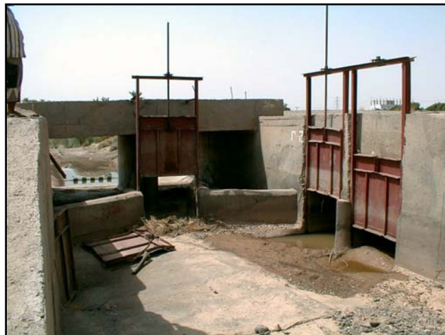
Cross Regulator, Beizag Main Canal 14 August 2002
