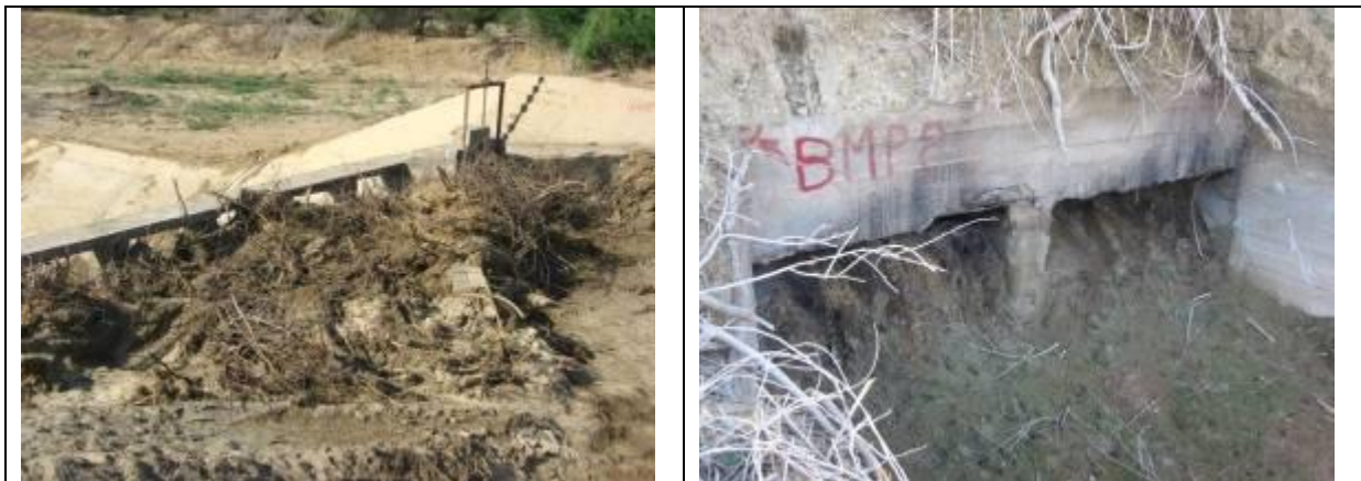
Excessive Siltation and Sediment Transport in Ahwar Due to Loss of Ground Cover
