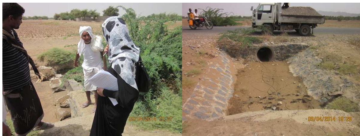
Figure 8.6: Left photo: the canal in which the soil bags are put to divert floodwater to Person 82's land. Right photo: channel that goes from the main canal to Person 82
