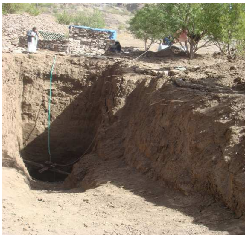
Figure 7.3: The higher well of 12m dug in farmer's field
