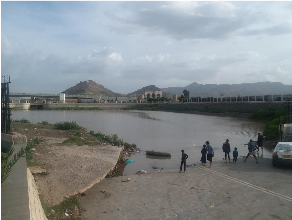
Figure (4.18): The retention pond of Al-Sabeen district filled with stormwater runoff
