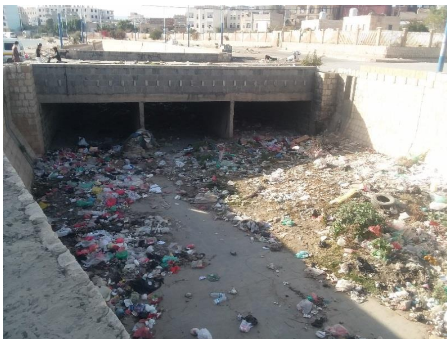
Figure (A6-12): Garbage dumps in main channel. This picture was taken by researcher in Al-Sabeen district
