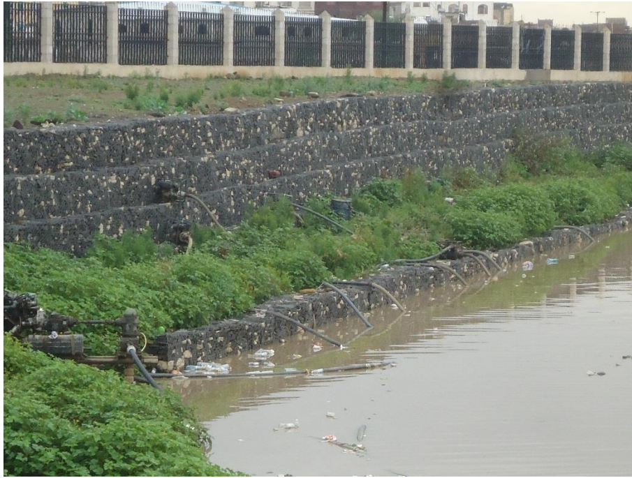
Figure (3.12): Water pumping from the retention pond at Al-Sabeen district into nearby farms
