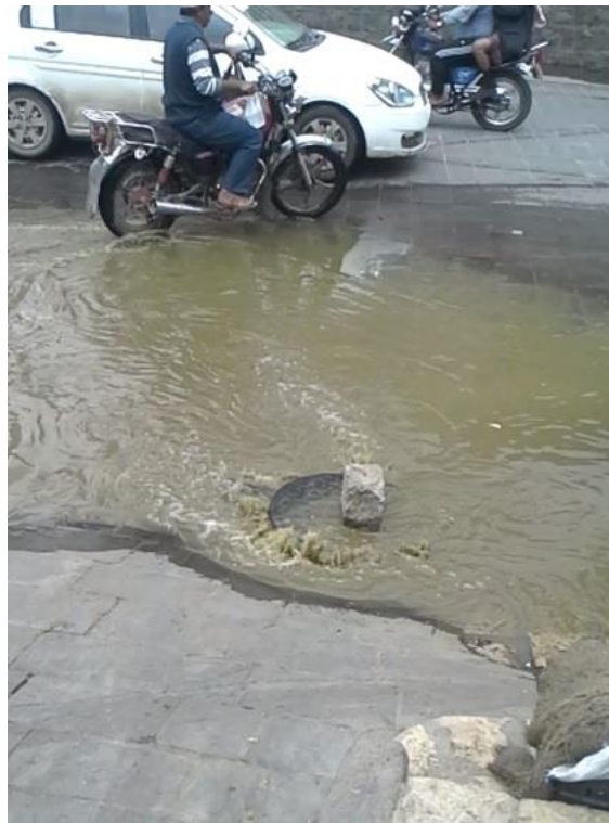
Figure (A6-10): The overflow of the sewage system in the Al-Saylah channel close to the old Sana'a city
