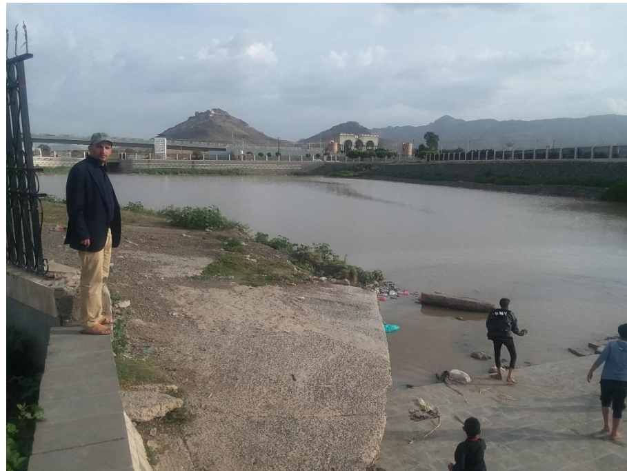
Figure (3.11): The stormwater retention pond in Al-Sabeen region at Sana'a city
