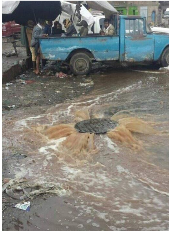
Figure (4.7): Overflow of the sewage system and mix up with runoff in Shuob region (Social Media Platform 2019)
