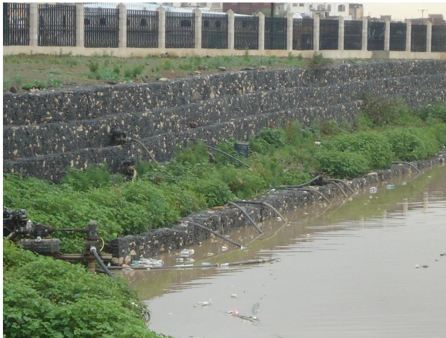
Figure (A6-8): Water pumping from the retention pond at Al-Sabeen district into nearby farms
