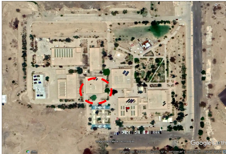
Figure (3.5): The rooftop of the Faculty of Engineering at Sana'a University-Reference site (Google Earth)
