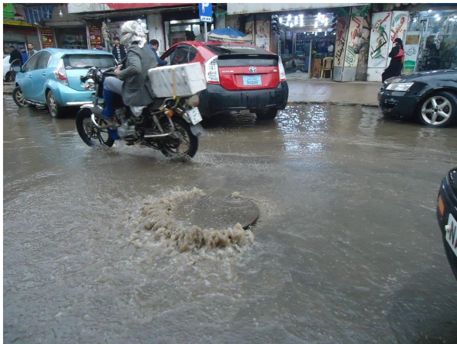
Figure (A6-6): Sewage system overflow Because rainwater has mixed with wastewater, this picture was taken in Tahrir Square during a rainfall event
