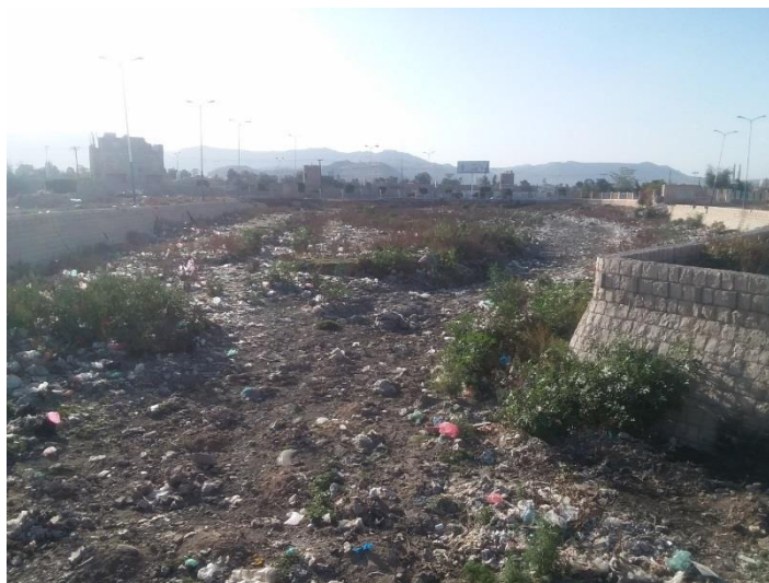
Figure (4.9) : Wastes and sediments in rainwater channel in Ma'ain district
