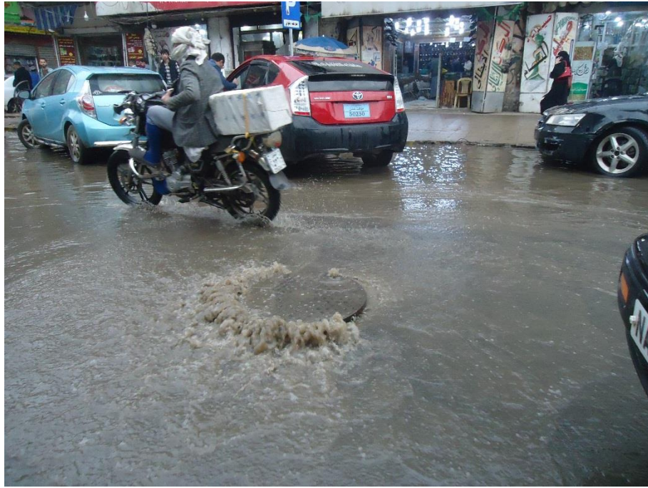
Figure (3.10): Sewage system overflow because rainwater has mixed with wastewater, this picture was taken in Tahrir Square during a rainfall event
