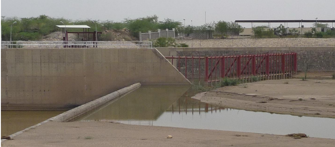
Figure 2-3: Barquqa weir trash screen at intake
