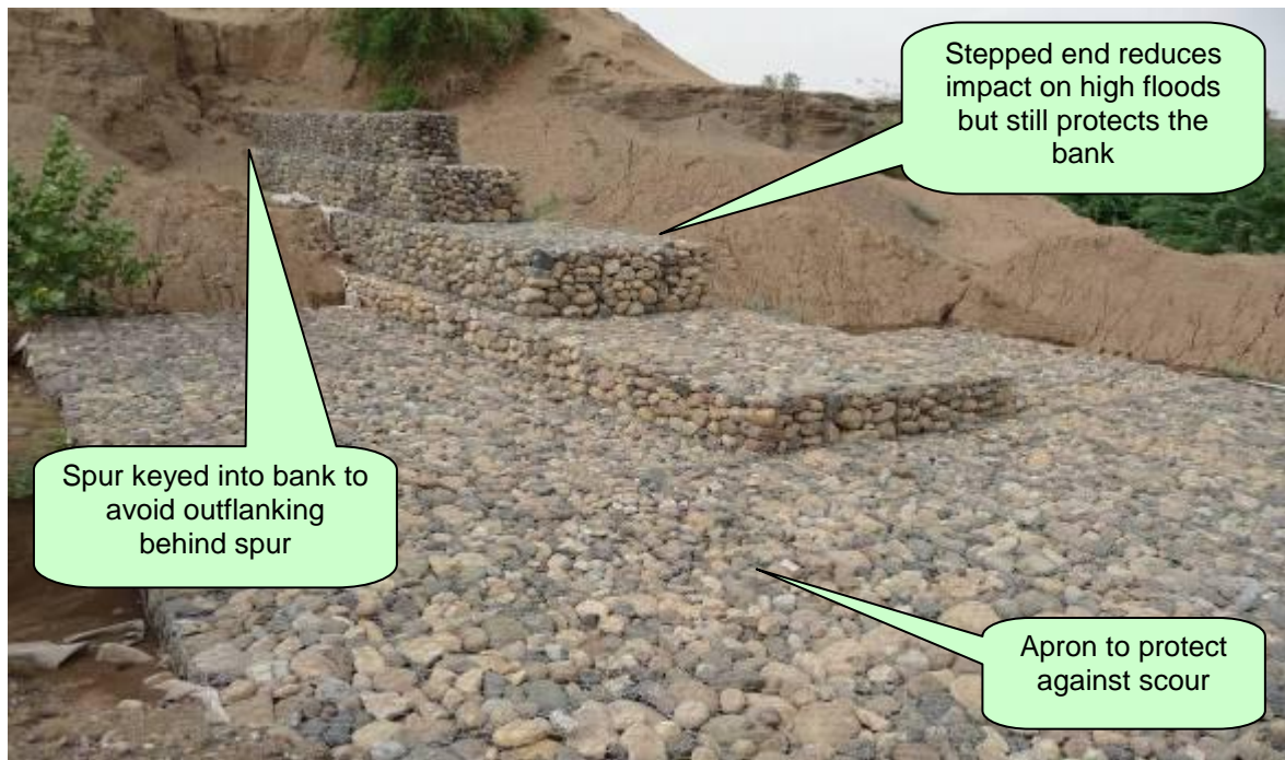
Figure 3-3: Generous scour protection at head of spur
