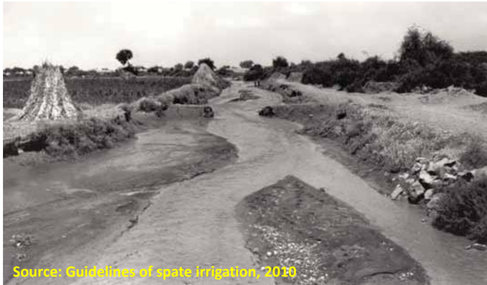
Picture 3.2 spate diversion under traditional system of wadi zabil
