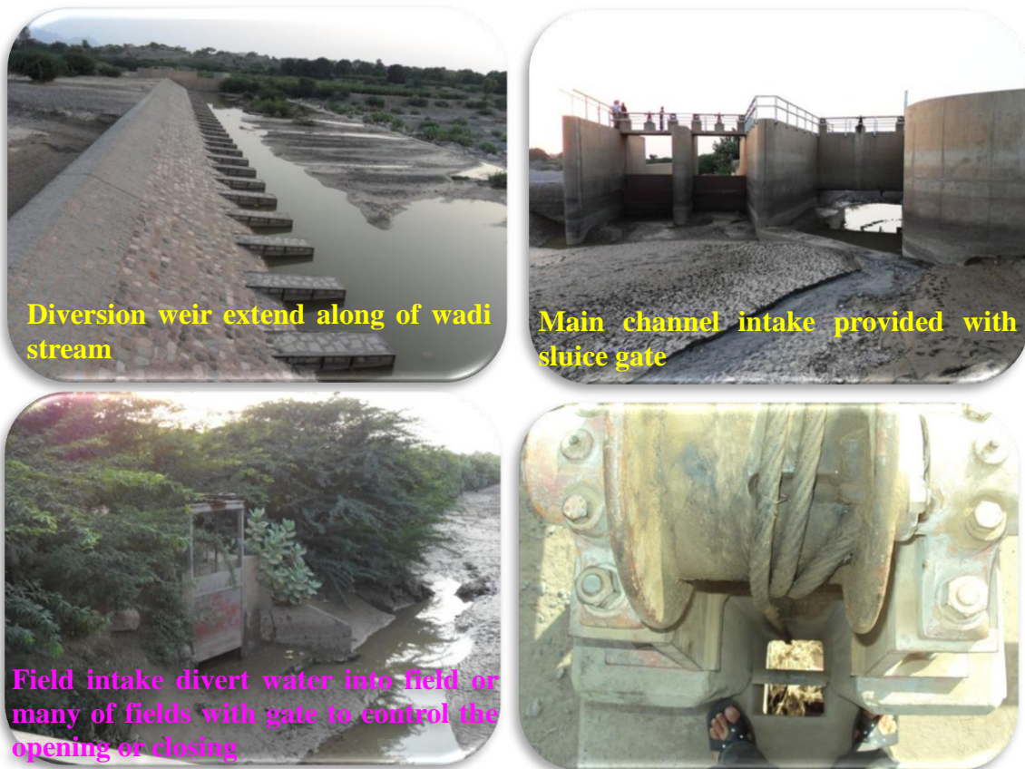
Picture 3.4 some components of modern spate irrigation scheme of wadi Zabid.
