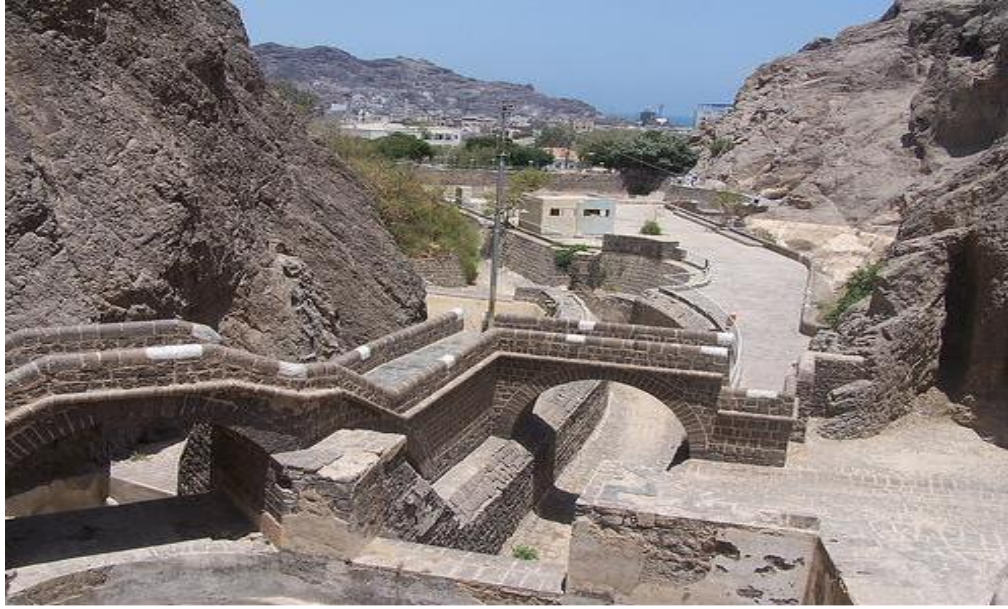
Figure 2-10. Tawila RWH tanks, Aden
