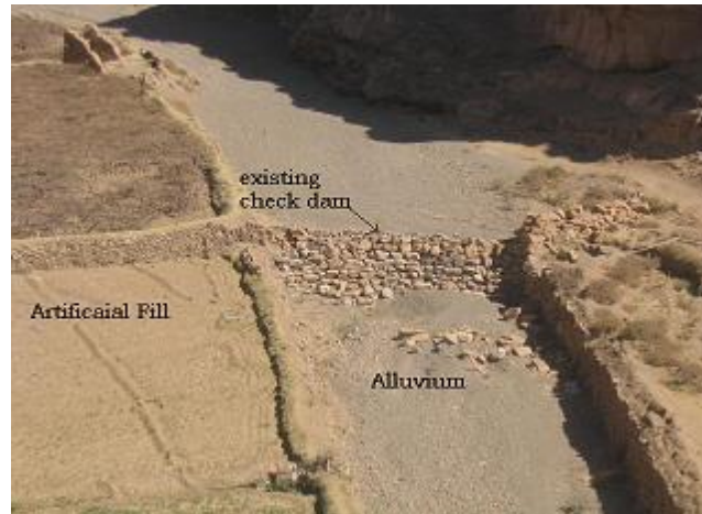
Figure 5 - 23. Downstream of Check Dam Area
