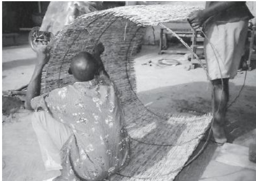
Figure B-1. Making the bamboo mat in a cylinder shape and reinforcing it with three circles of steel wire
