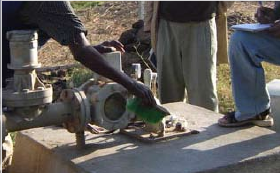
Installing a deep tube well, Ethiopia
