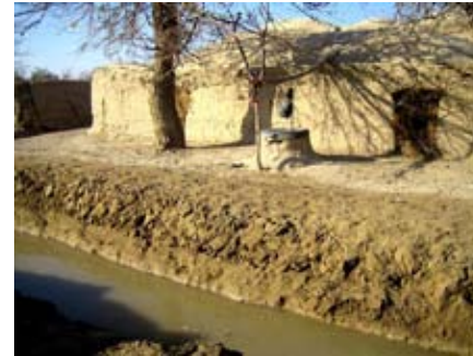
Wells constructed next to irrigation channels in areas with saline groundwater. The wells tap the seepage from the irrigation canals that is less salty, Afghanistan
