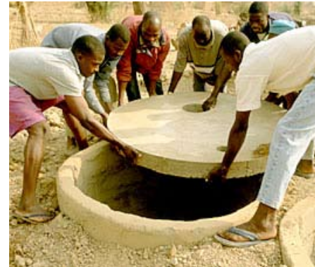
Building a Ventilated Improved (VIP) latrine in Ghana
