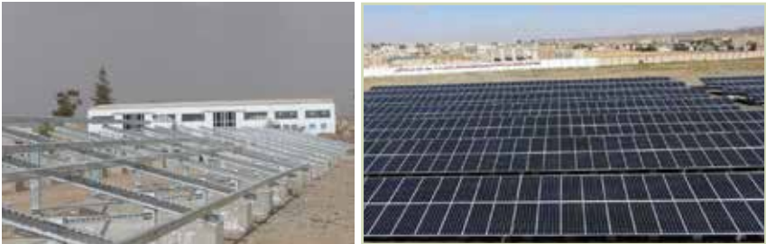
Figure 15 Installation of solar panels
