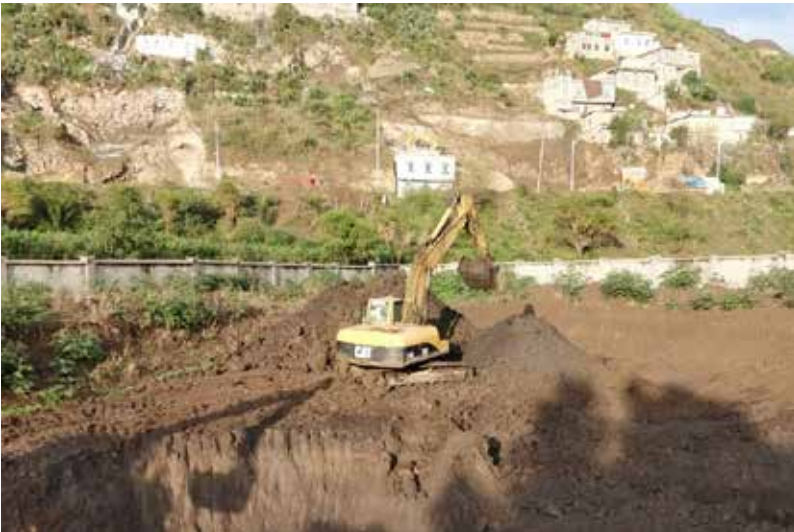
Figure 29 Ponds during construction and operation
