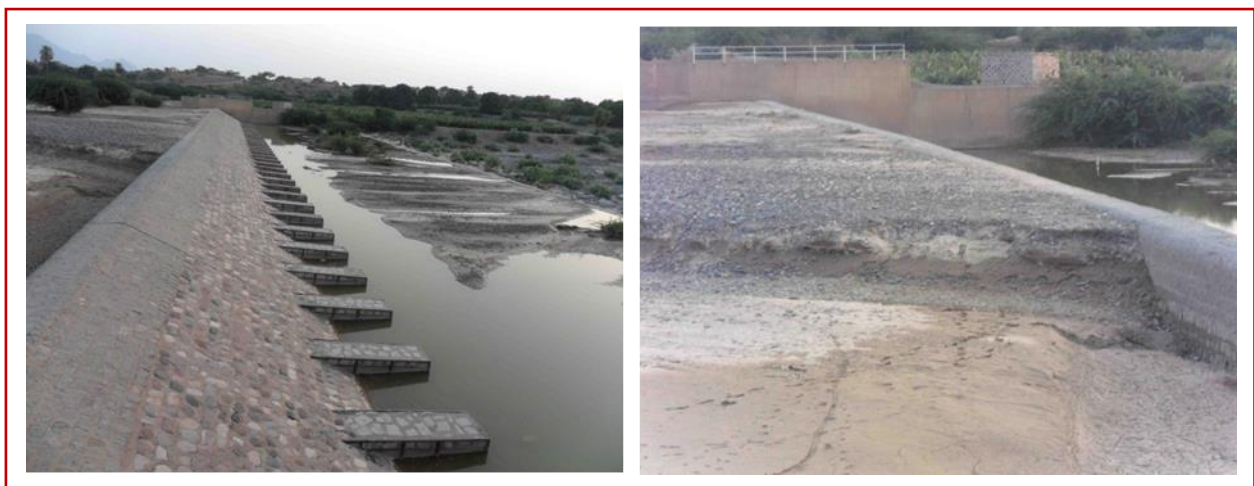
Figure 2.7: Photos shows the raised body of weir 1 and the current sediment accumulation.
