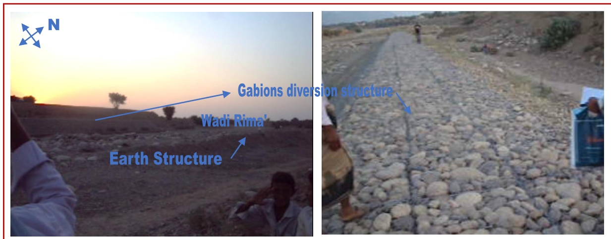
Figure 2.6: A: the constructed gabions diversion structure in the southern side of wadi Rima'a, and the earth diversion structure in North side of the wadi.
