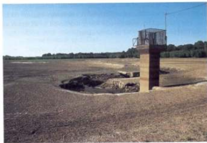
FIGURE 10.15 This dam is now useless because its reservoir has filled with silt and sediment.
