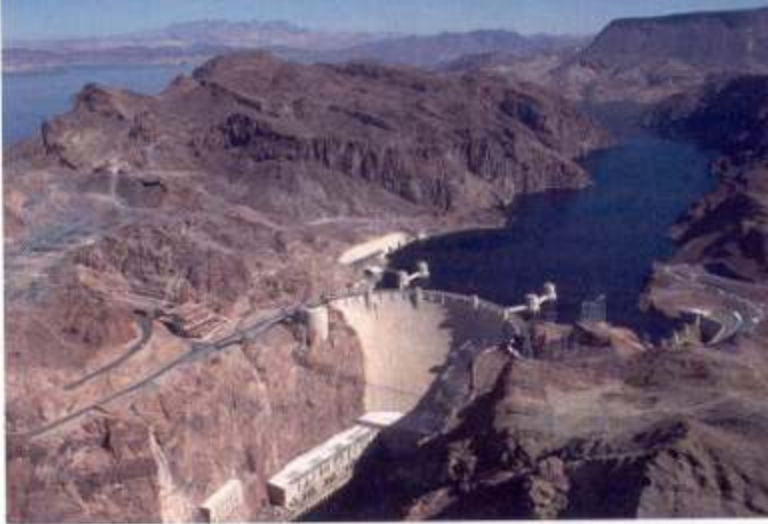
FIGURE 10.14 Hoover Dam provides valuable electric power to Nevada and California but Lake Mead, behind the dam, loses about 1.3 billion m 3 of water per year to evaporation.
