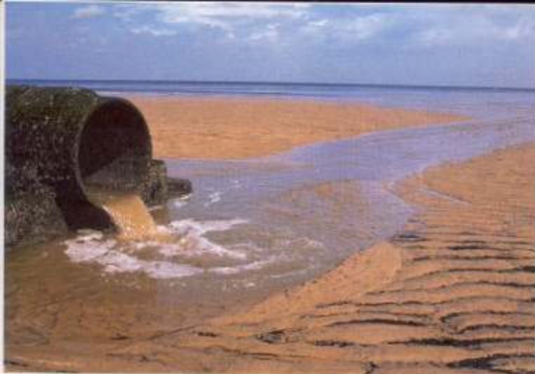
FIGURE 10.18 Sewer outfalls, industrial effluent pipes, acid draining out of abandoned mines, and other point sources of pollution are generally easy to recognize.
